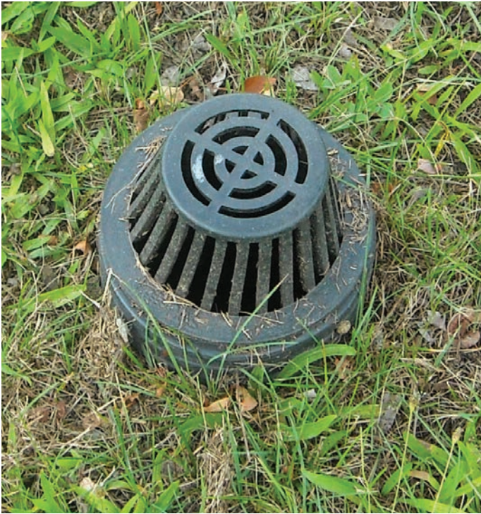
Figure 57. Rainwater basin drain.
