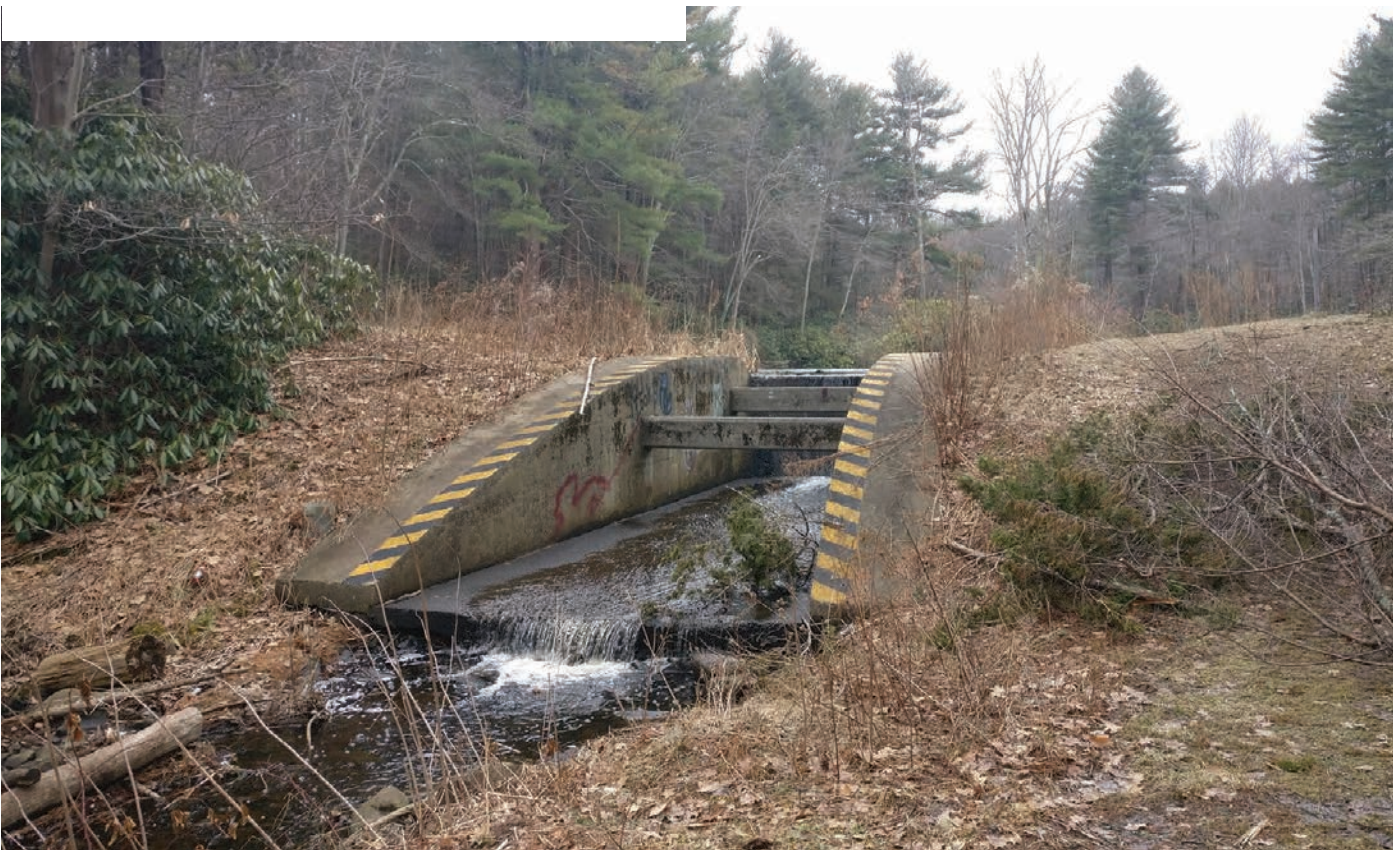
Figure 44. Pond Spillway within Cochran Sanctuary.
