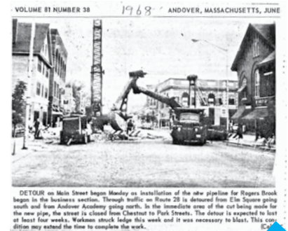
1968 Rogers brook was put underground. A large trench was dug through the center of the park to place a six-foot conduit.
